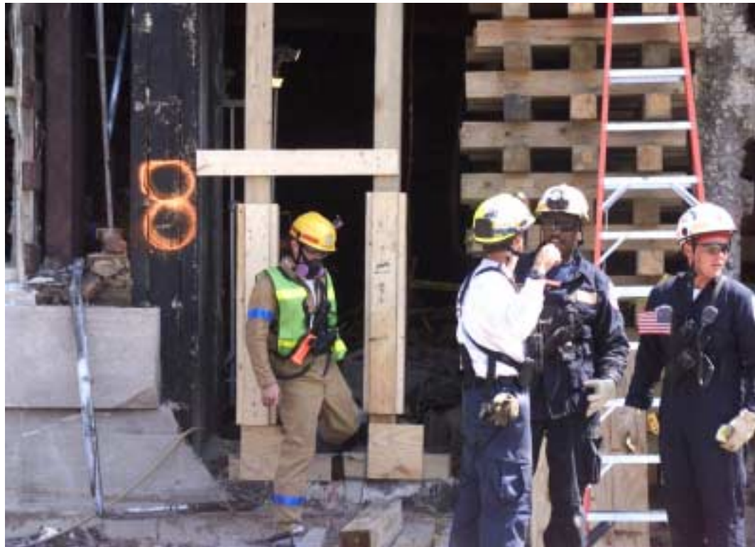
US&R shoring and marking system.
